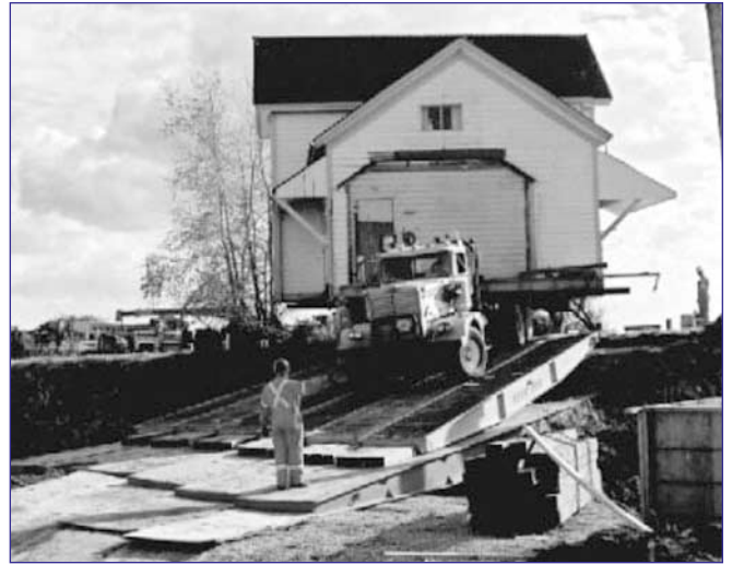
Negotiating the perilous right angle turn down the ramps
