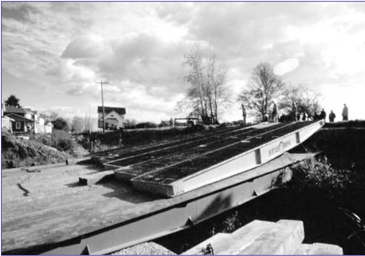
Ramps used to bridge the dyke
