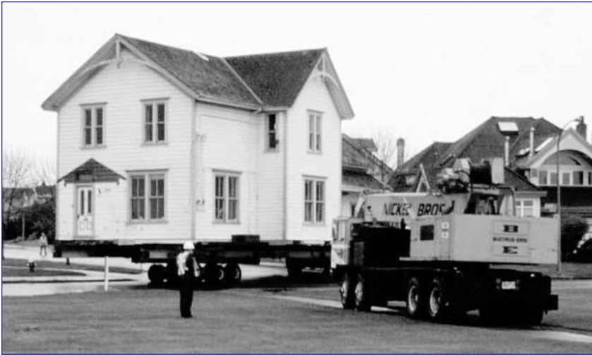
Jockeying the house onto the grass towards the barge
