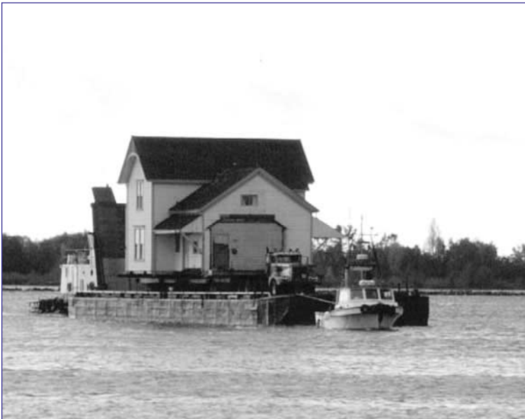
Transporting the house by barge in Steveston Channel
