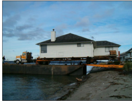
This 3-bedroom house near Mutiny Bay in Freeland is loaded onto a barge to be transported to Everett. An Everett company recycles unwanted houses, saving money and the waste of tons of building materials.
